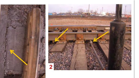
1: It may be necessary to chip away compacted snow and ice off the tie plate to get the switch to latch and get a switch point that does not gap.
